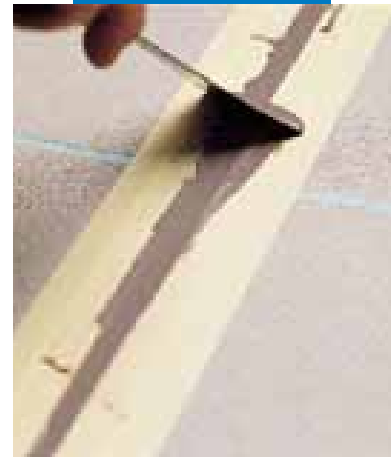
Smoothing the joint
