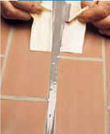
Expansion joint in red quarry tile floor sealed with Mapeflex PU21
