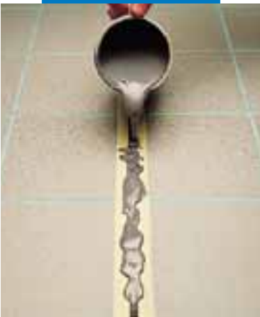
Filling the joint with Mapeflex PU21
